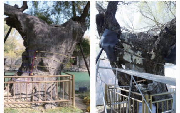
图 13 古柳 L03 修复前后对比 Fig. 13 Comparison of pre-repair and repair of L03
